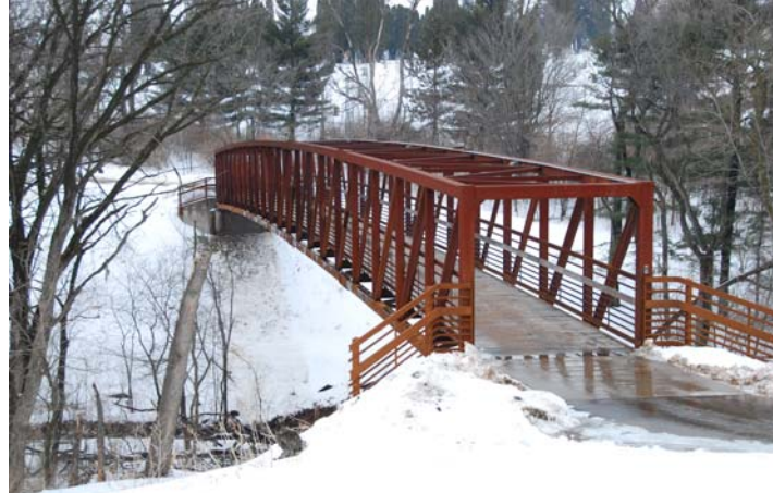
Figure 20: Box Truss Bridge
