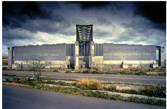
Figure 2: Solid Waste Facility Exterior
